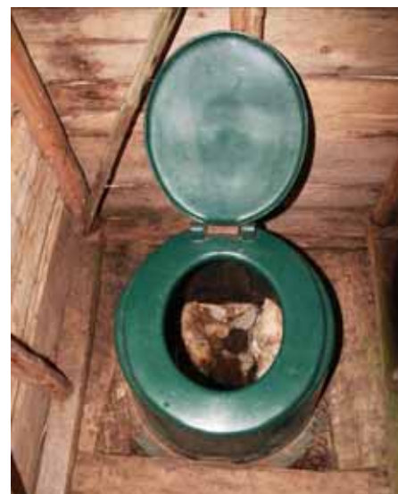
✘ Hole in floor not big enough!
