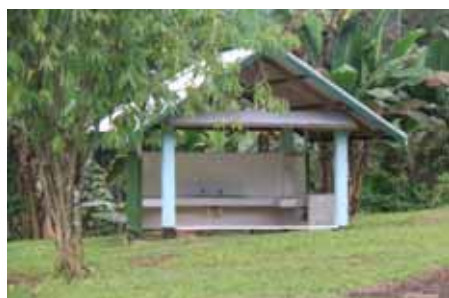
✓✗ Plumbed, tiled, sink in a cooking house, Kavelo.
