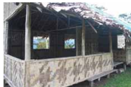
✓ Seat under eave allows boot putting on/removal out of rain, keep mud outside.
