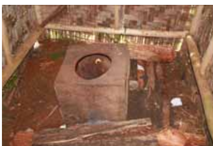
✗ Rough timber pedestal.
