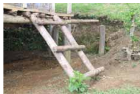
✘ Round steps in a ladder form, difficult for many trekkers to use.
