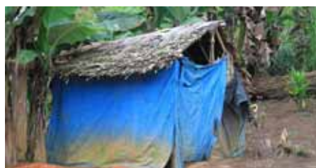
✗ Need better walls than plastic, can use bush materials.
