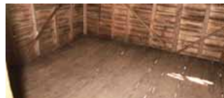
✓ Timber external cladding. Timber floor, nails need to be punched or they may puncture trekker's inflatable mattresses.
