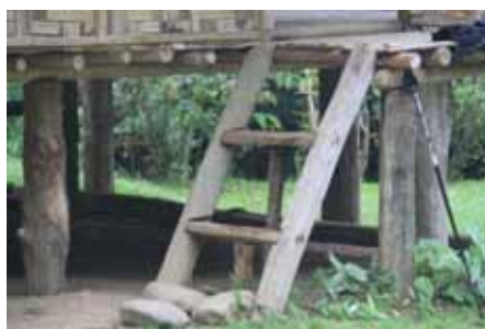
✓* Steps a bit too steep, but otherwise, good landing stones, good height and good tread/step width.
