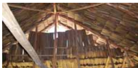
✓ Offset, but overlapping thatching on gable ends, allows ventilation but keep rain out.
