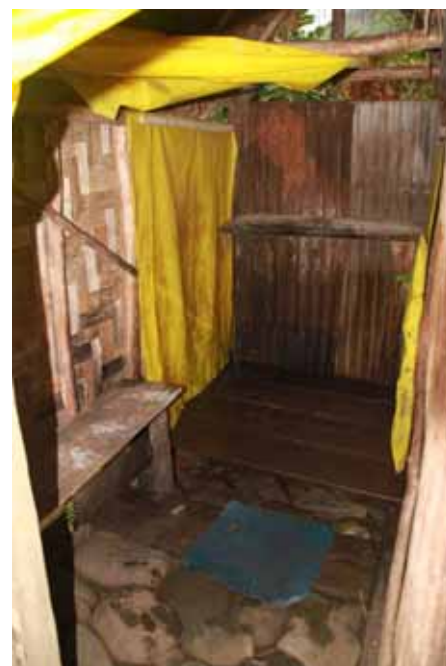
✓ Looking inside, seat to put towel, clothes and change. Well drained rocks in outer area and timber grate on shower floor. Inner shower curtain. Soap/shampoo shelf.
