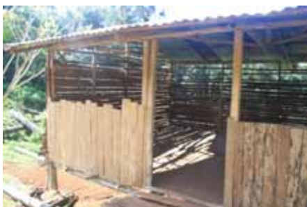
✓ Different wall cladding, split timber and saplings.
