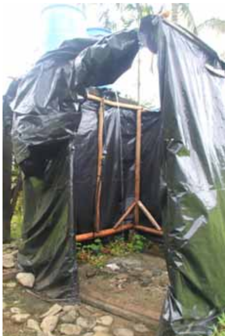
✗ Reasonable design, black plastic could be replaced with woven mat or bush saplings.
