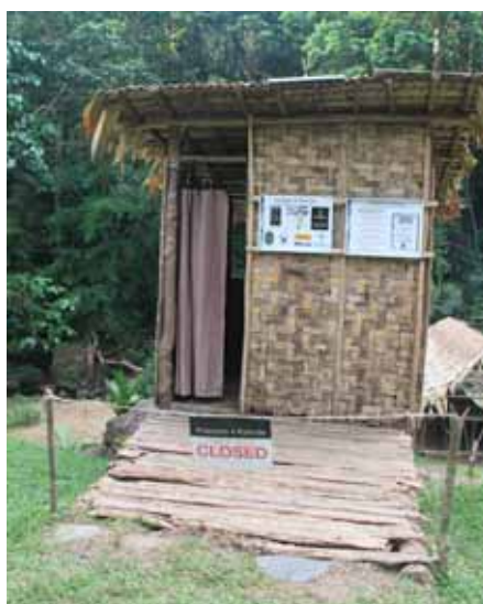
✗ .Good composting toilet, but maintenance needed.
