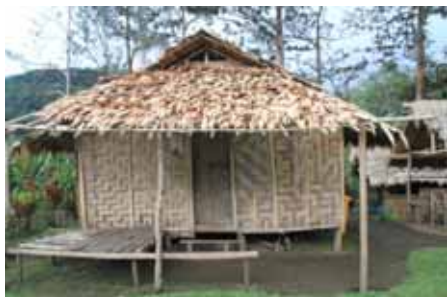
✓ Covered platform near door allows backpack, boot and rainwear removal in rain.
