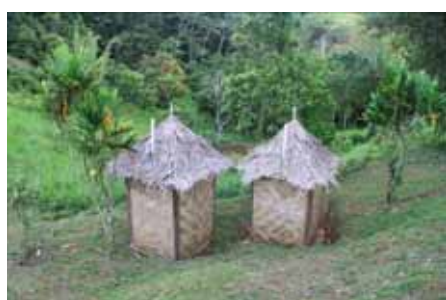
✓Good pit ventilation.
