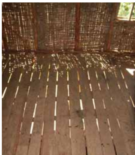
✓✘ Woven sapling wall, neat bush planks floor. OK for Trekkers hut, not for guesthouse or lodge.
