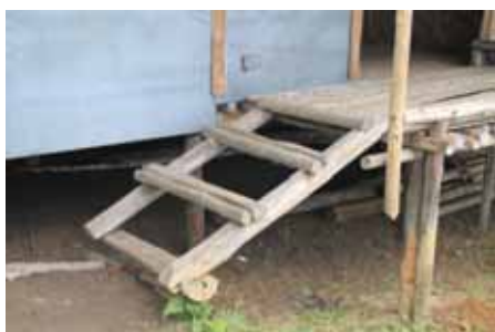
* Angle a bit too low and steps uneven with no flat surface make these difficult to use.
