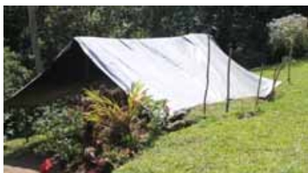
✓✘ Tarpaulin roofed dining house.
