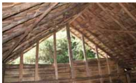
✓ Open gable with long roof overhang allow ventilation and keep out rain.
