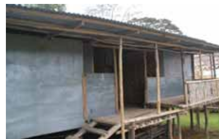
✓✘ Galvanised sheet used for wall cladding, unsightly, but durable.
