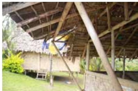
✓ Neat bracing of overhanging eaves.
