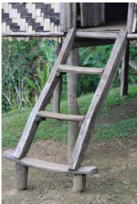
* Bottom step uneven and moves, steps too far apart (in height) and a bit narrow.
