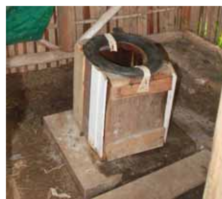
✗ Rough timber pedestal.
