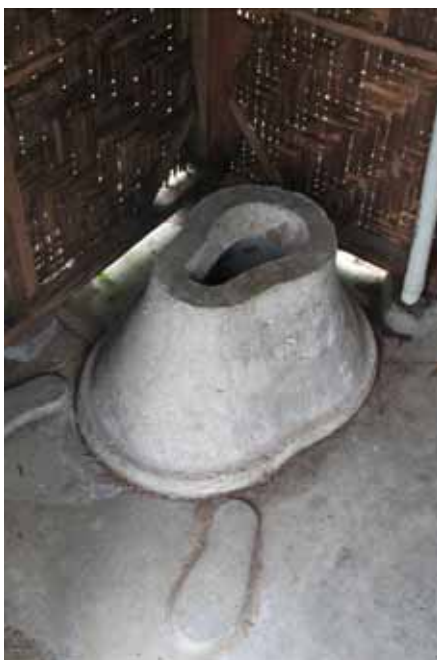
✗ Concrete moulded base and pedestal. Very difficult for trekkers/tourists to use. The hole is set back from the base and difficult to squat above. The "feet" are not located in placed in located most trekkers can put their feet!
