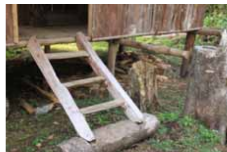
✘ Step height uneven, top step mismatched and not level with floor. Middle step very narrow. These factors make this step a safety concern.
