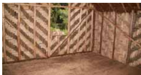
✓ Very neat wall cladding and floor.
