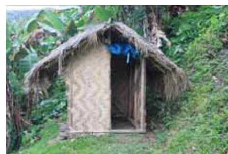
✗ .Door too narrow, no ventilation and only plastic sheet door.
