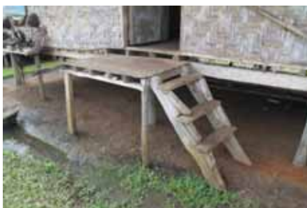
✓✘ Steps with landing, top step height mismatched to landing height (not an even spacing) and needs a handrail.
