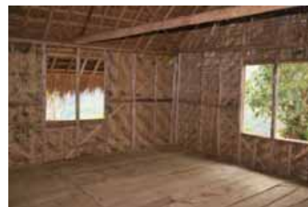
✓ Large open floor typical of trekker hut.
