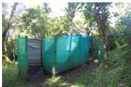
✓ Shade cloth used to effectively screen shower, area inside for dry separate changing area and shower area.
